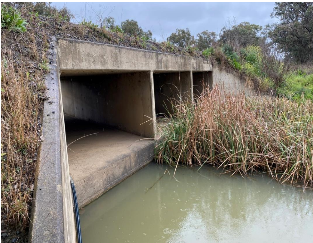
Figure 2 – Culvert 3 existing arrangement.
